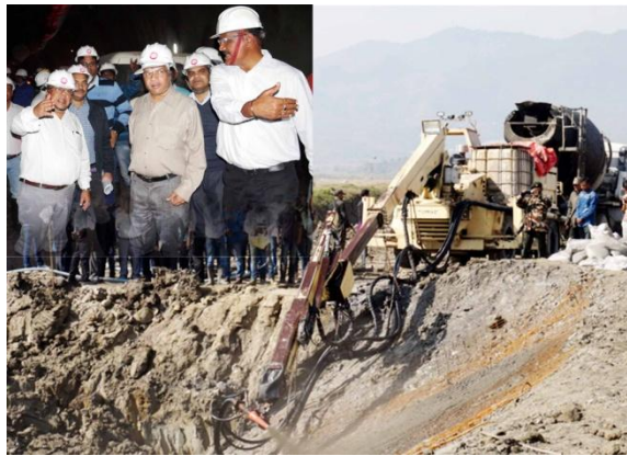
Shri N.K.Prasad, GM/Con, N.F.Railway & other Sr.Officials at Tunnel construction site on 19.12.2017
